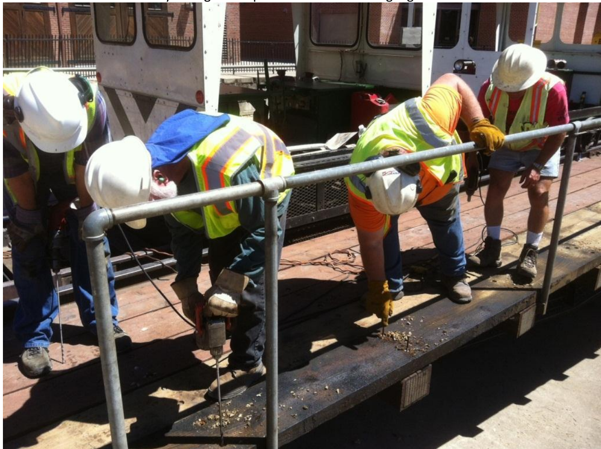
The MOW Drill-Team (Steve N., Mike M., Frank, and Steve M.) installing the final deck-plank.
