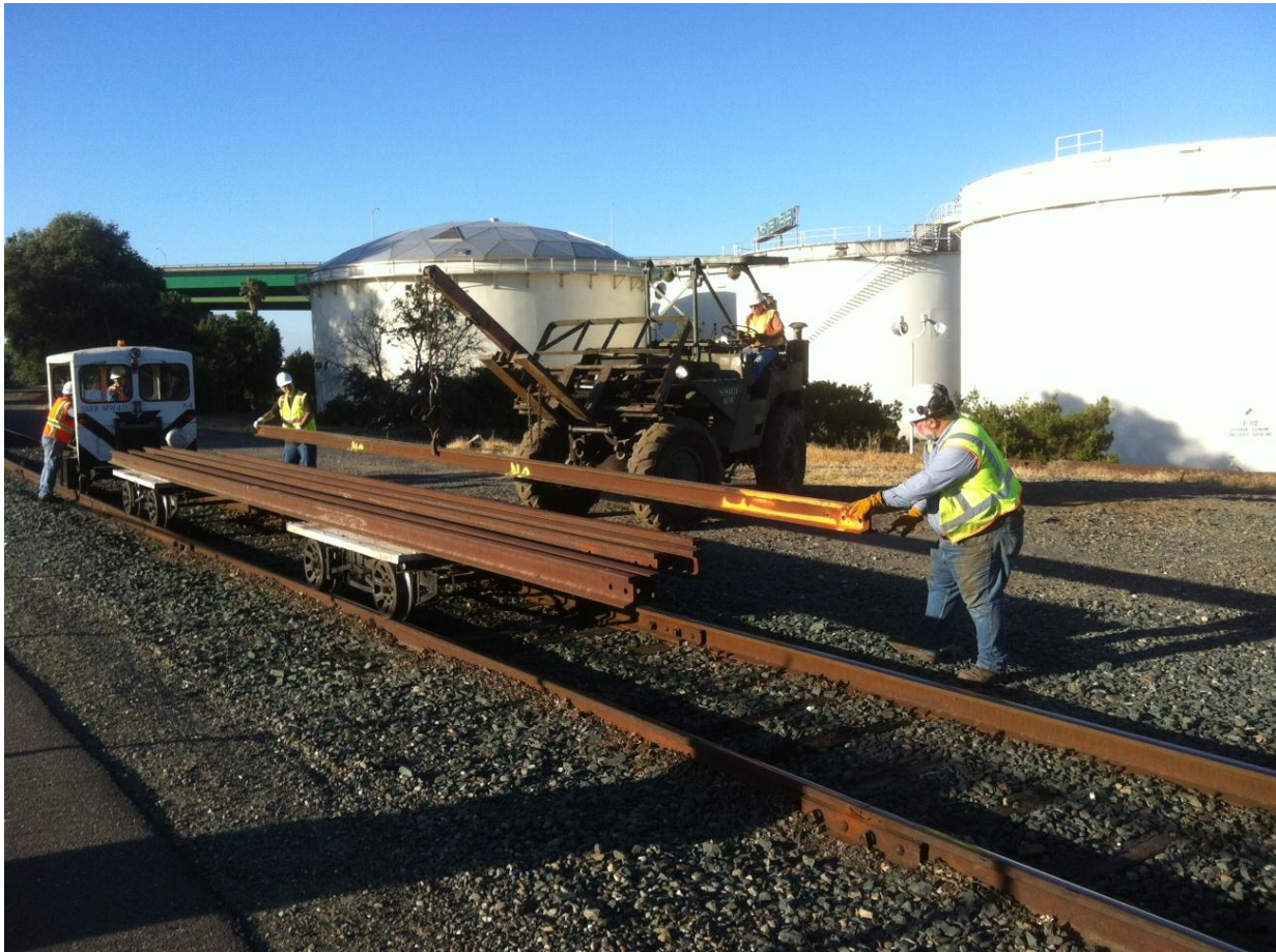
Mike on Big Green while Brian and Frank guide a stick of rail onto the flat cars.
