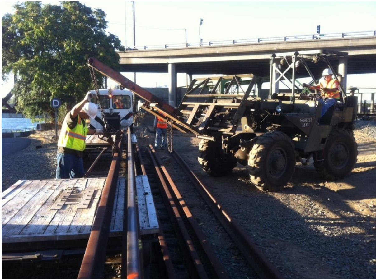
Brian and Mike unloading rail along the old Track 150.
