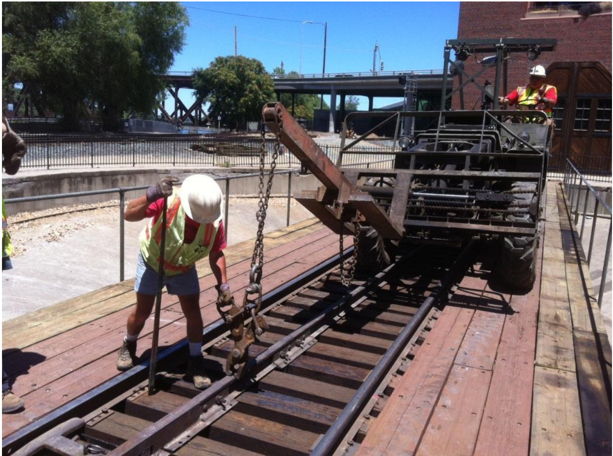
Steve M. and Harry on Big Green place the west narrow gauge rail on the turntable.
