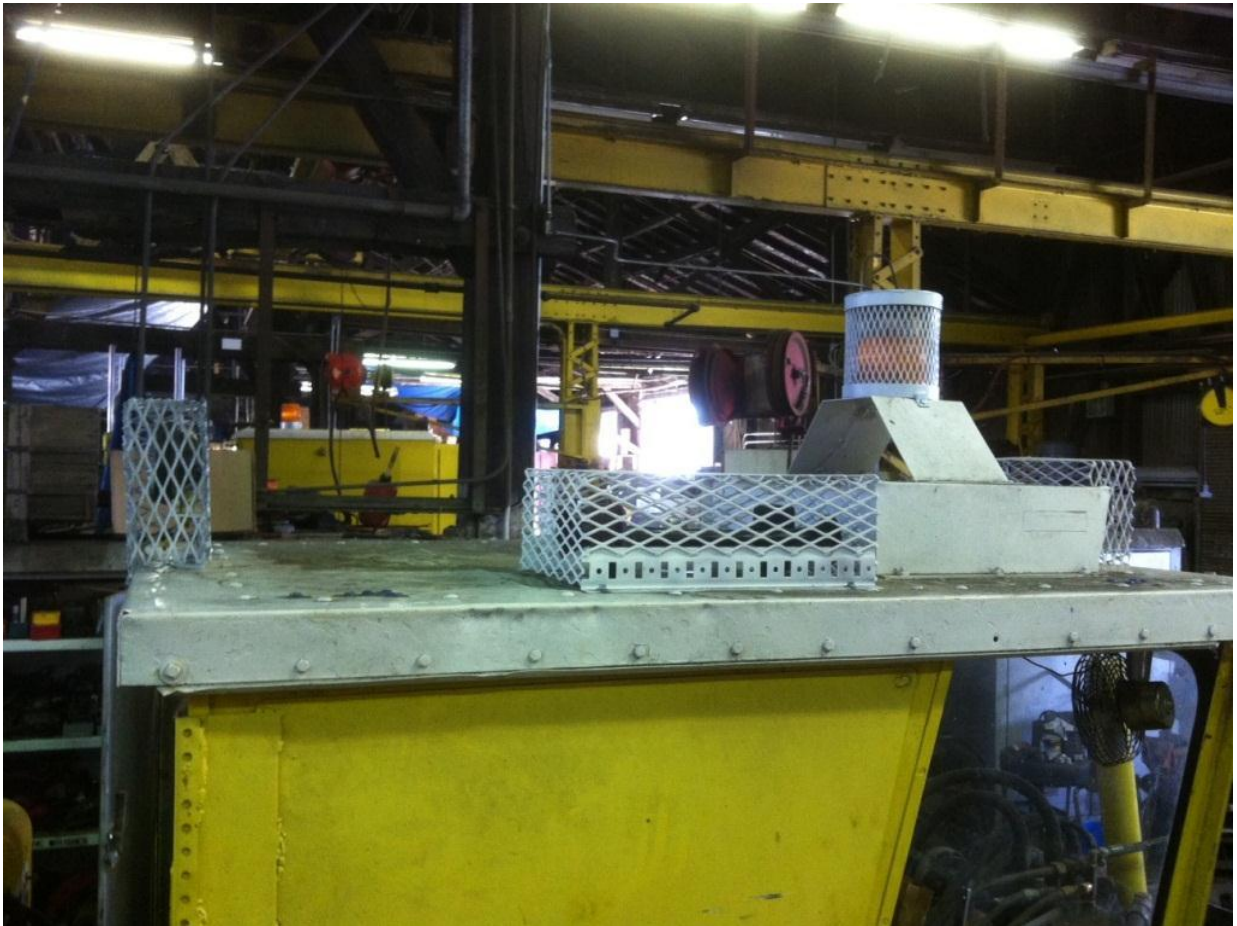
Cliff's artisanship on anti-vandalism shields for the scarifer-inserter.
